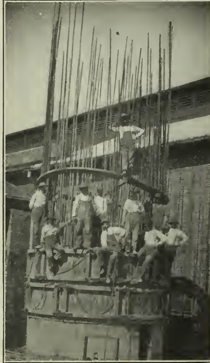
FIG. 1. METHOD OF REINFORCING CONCRETE STACK
